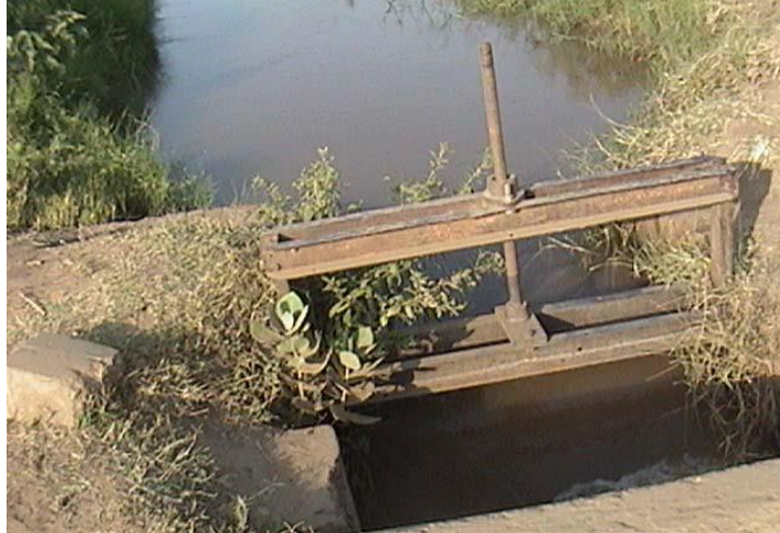
Fig. 5. Weeds and silts at movable weir opening (1.3m)
